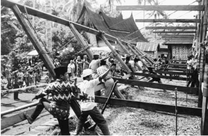
3.7 Raising the framework of small posts, Bakah Dalam, 1996. Photo: Marcel Vellinga.
