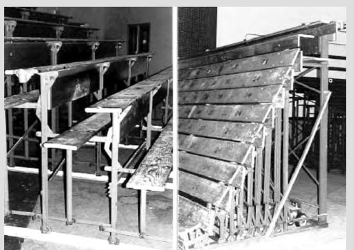
**Figure 25.42** Manually operated telescopic bleachers (above) may collapse if not operated properly (CPSC, 2001).
