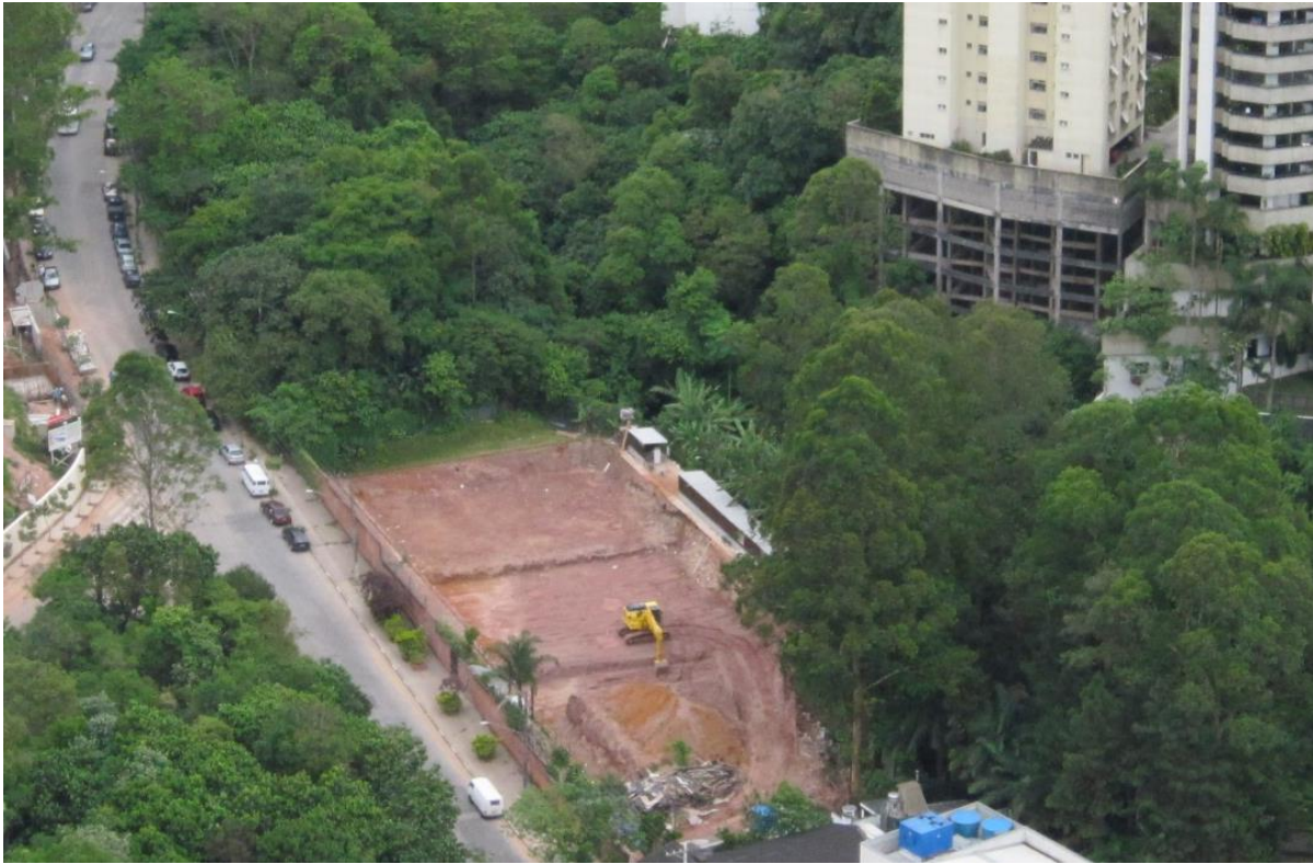
Authorized vegetation clearance for urban development
