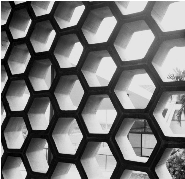
FIGURE 2. Cobogó panel in the school building, c. 1950. Source: Centro de Documentação Syvio de Vasconcelos, UFMG.
