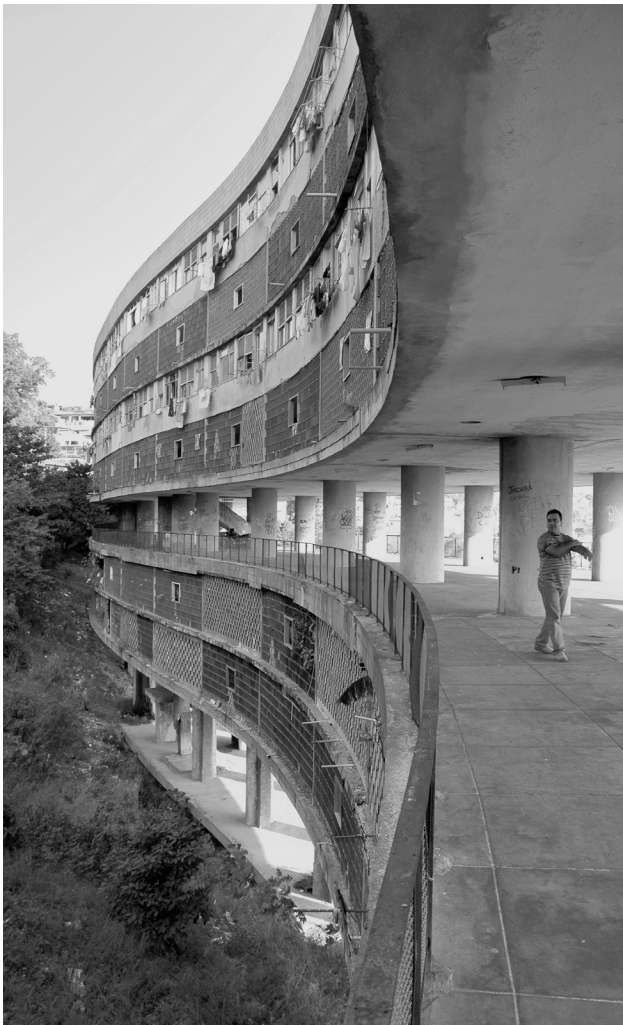
FIGURE 15. Block A, showing the cobogó facade and the intermediate level, c. 2000s. Source: Pioneers of Social Housing Archives.
