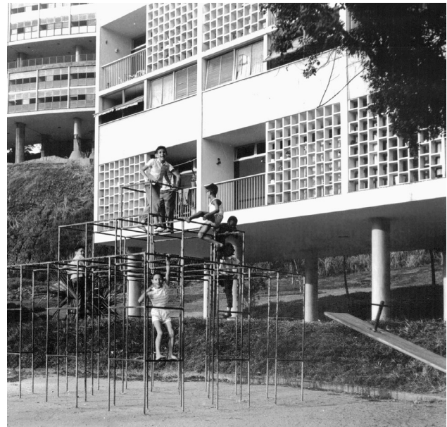
FIGURE 13. Playground area next to Block B apartment building, c. 1950. The cobogó panels can be seen. Source: Arquivo Geral da Cidade do Rio de Janeiro.
