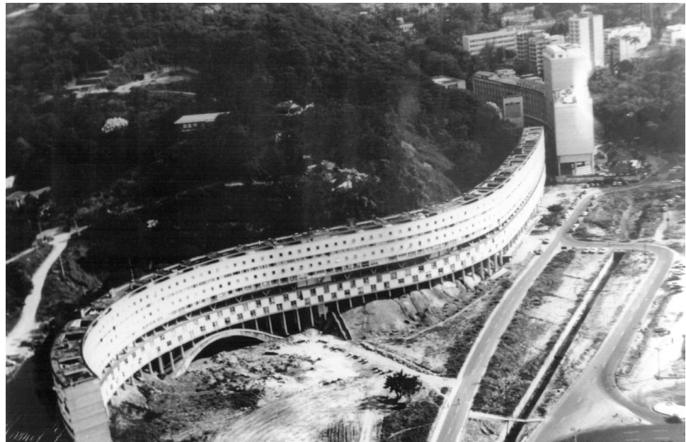
FIGURE 6 (RIGHT). Marquês de São Vicente Housing Complex in the South Zone of Rio. The former favela and provisional proletarian park in front of it had just been removed, c. 1960s. Source: Arquivo Geral da Cidade do Rio de Janeiro.
