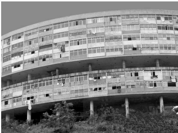
FIGURE 17. Block A before renovation, showing how most of the windows had already been changed by the residents, 2004. Photo by author.
