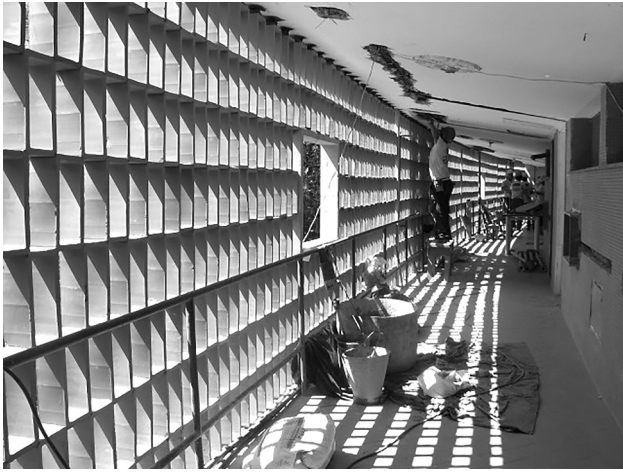
FIGURE 19. Block A apartments corridor, showing a new cobogó panel in the process of being assembled, 2015. Photo by Alfredo Britto.
