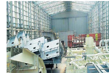
The indoor painting shops are where hull blocks are painted. The controlled ambient conditions, improve painting quality.
