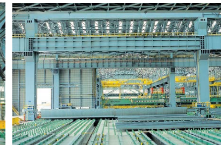
A high indoor PE (pre-erection) site can produce 40 m long blocks inside the panel shop. Additionally, all pre-outfitting work can be done indoors, making the site a virtual all-weather shipyard.
