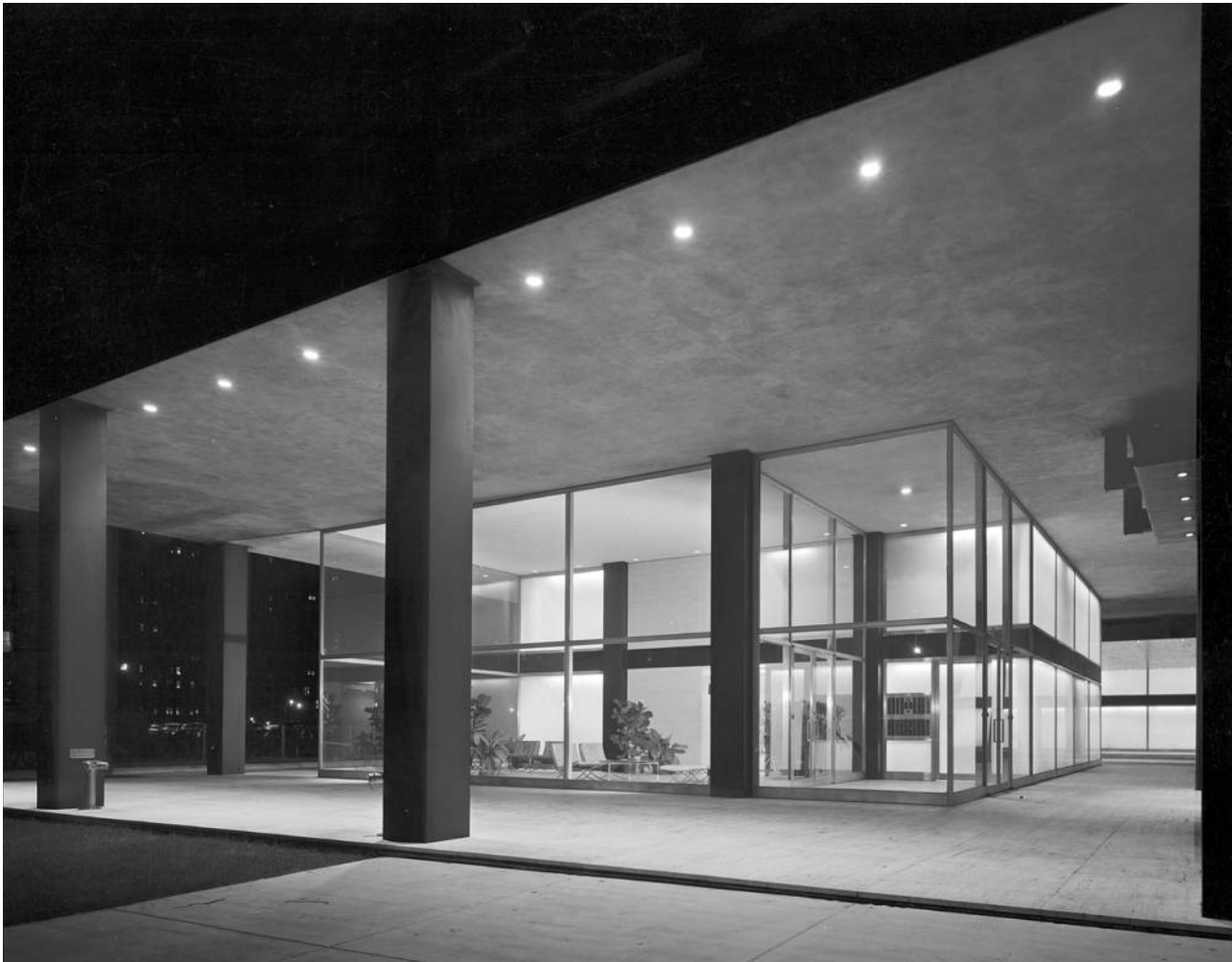
Figure 11 860–880 Lake Shore Drive Apartments, night view of glowing core and lobby
