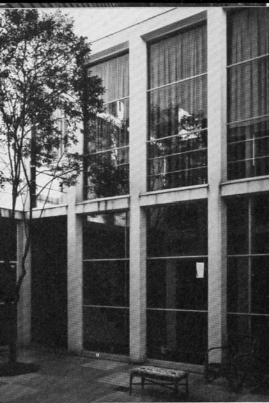
Frontini House, rua Monte Alegre, 957, São Paulo Bernard Rudofsky, architect, 1940-1941
