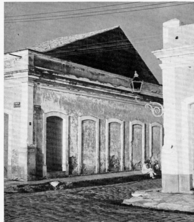
Old warehouse in Recife
