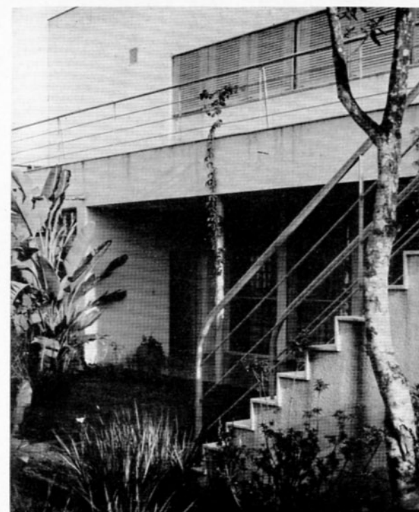
Courtyard of the Frontini House, São Paulo
