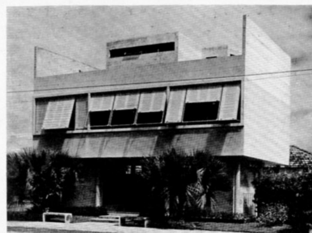
Push-out, roll-up wooden blinds in metal frames shade de Brito's Anatomical Laboratory in Recife
