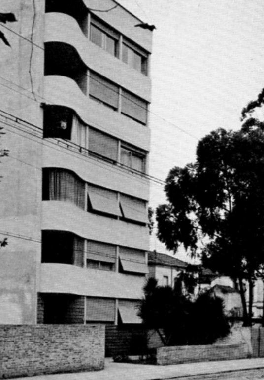
Apartments, Alameda Barão de Limeira, 1003, São Paulo Gregori Warchavchik, architect, 1940
