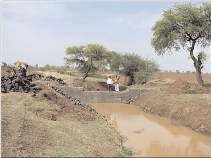
FIGURE 7.3 Check dam: work is completed.
