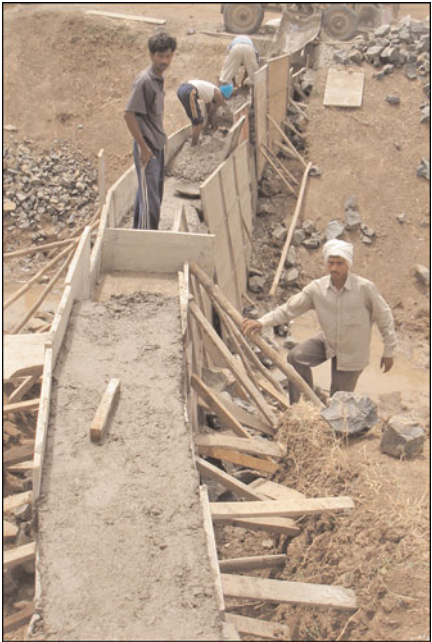
FIGURE 7.2 Check dam: a work in progress.
