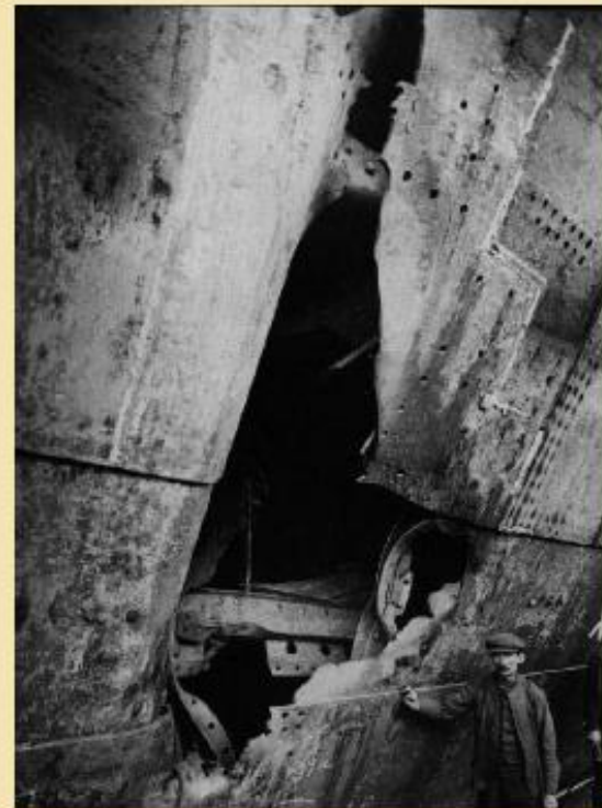
Hull of the Olympic , Titanic 's sister ship after a collision in 1911.
