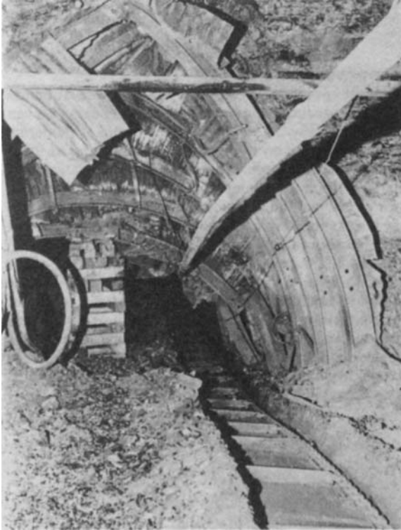
Fig. 16.18 Partial closure of an originally horizontal main road (courtesy of the National Coal Board, London).
