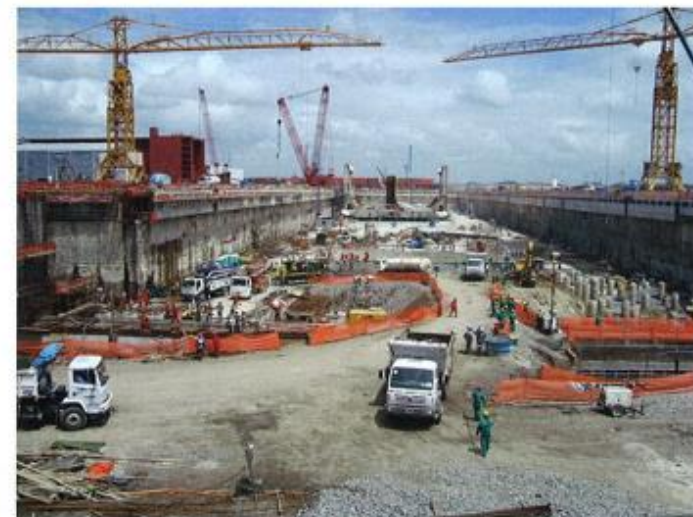
Construction underway for the dock floor
