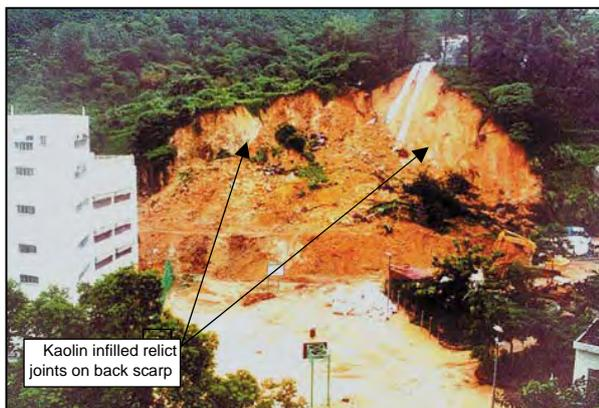
Figure 6.4.22 – 1995 Fei Tsui Road landslide
