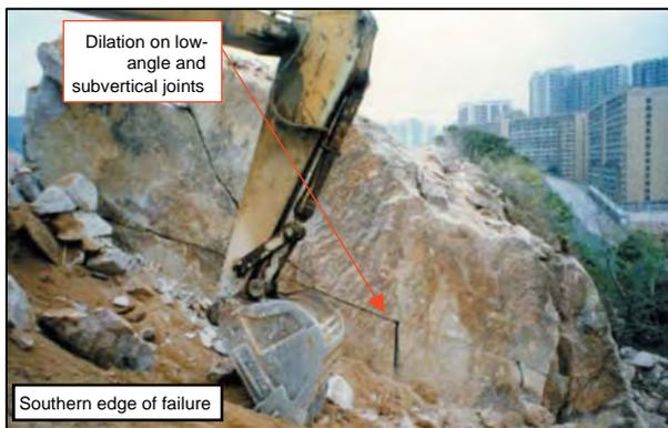
Figure 6.3.4 – Blast-induced failure during site formation works at Sau Mau Ping Road in 1997 (Leung *et al.*, 1999)
