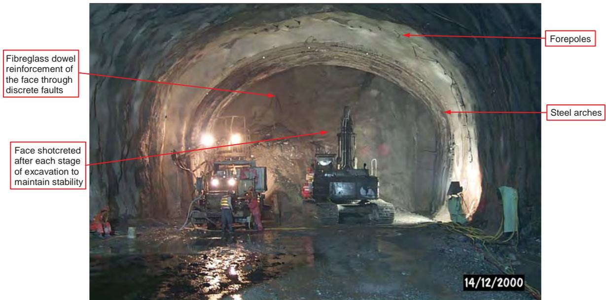
Figure 6.7.11 – Full face excavation, face reinforcement and forepoling during construction (photograph by Nishimatsu-Drageges Joint Venture)
