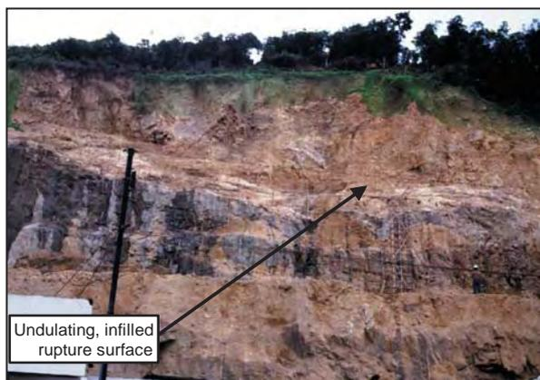
Figure 6.4.19 – 1982 South Bay Close landslide scar (Hencher, 1983b)
