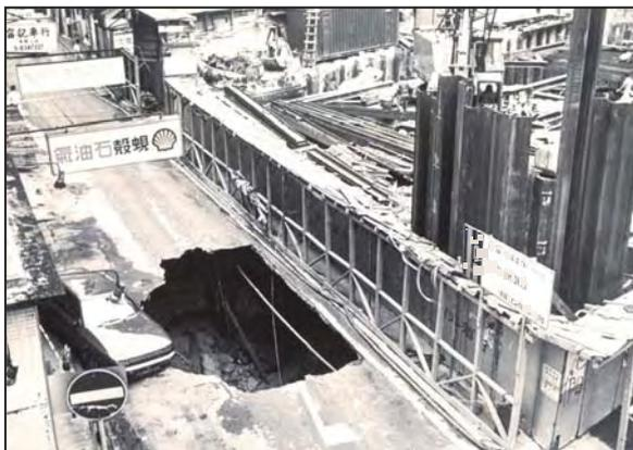
Figure 6.6.1 – Collapse of road due to boulders preventing adequate embedment of sheet piles retaining adjacent excavation
