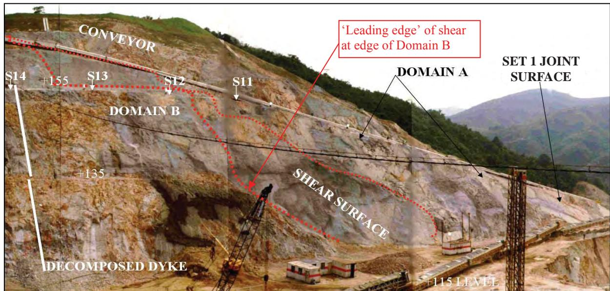
Figure 6.4.34 – Upper part of face during construction showing shear surface and Domains A and B (photograph by J.W. Tattersall)
