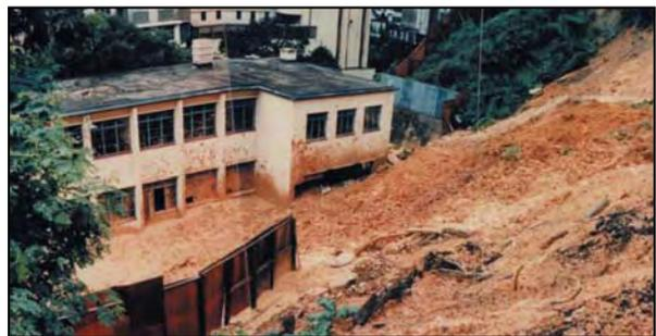
Figure 6.4.8 – 1988 landslide at Island Road School (Irfan, 1989)
