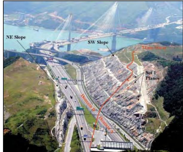
Figure 6.4.35 – View of completed cutting showing trace of main shear and Domains A and B
