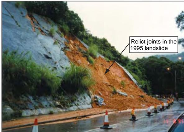
Figure 6.4.13 – 1995 landslide at Sai Sha Road with relict joints (Wong, 1997)
