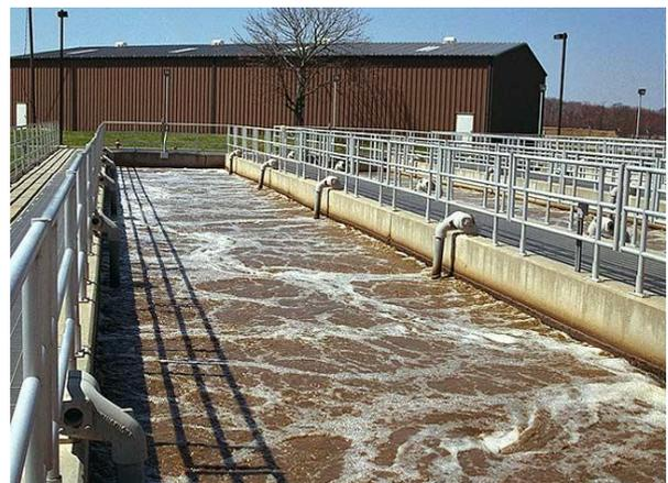
Fig.6. The bio-aeration tank<sup>16</sup>
