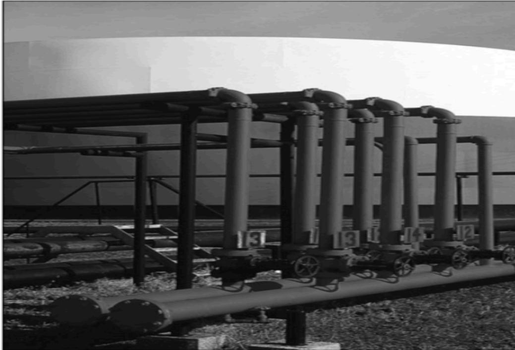
Steam pipe bridge in a geothermal power plant. Pipe flows are everywhere, often occurring in groups or networks. They are designed using the principles outlined in this chapter. *(Courtesy of Dr. E. R. Degginger/Color-Pic Inc.)*
