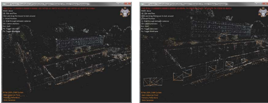
FIG. 11: The reconstructed sparse scene of Student Dining and Residence Hall construction project in Champaign, IL. The right image represents 7 camera frusta for which their images were used for sparse reconstruction of the as-built site.
