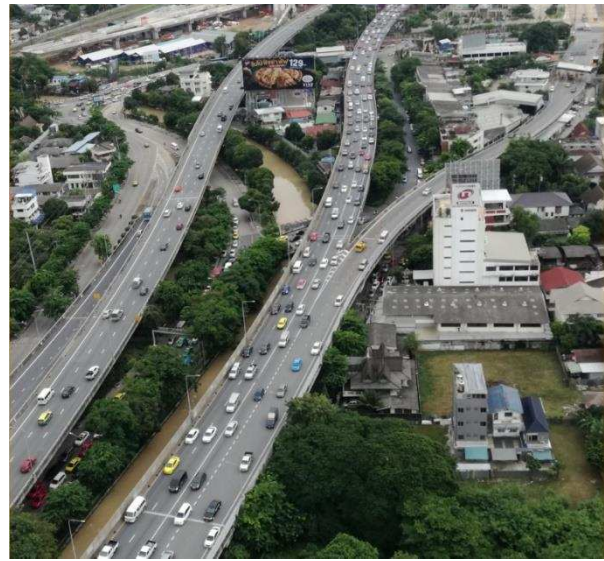
Figure 9: Shoulder lane driving on Sirat Expressway
