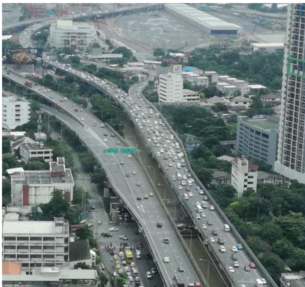
Figure 10: Shoulder lane driving on Sirat Expressway
