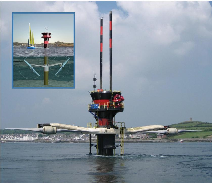
**FIGURE 3.42** A SeaGen turbine installed at Strangford Lough. (Courtesy of Seaflo and SeaGen Turbines, Marine Current Turbines Ltd., available at: <http://www.marineturbines.com>, March 2008.)
