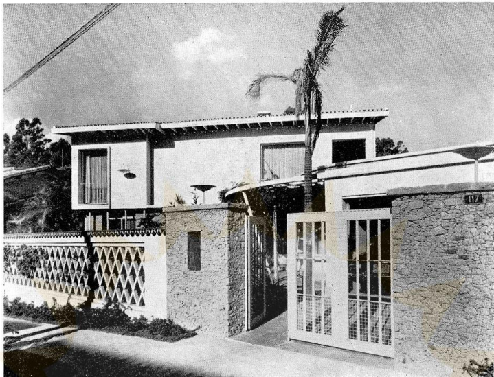
FACHADA PRINCIPAL COM GRADIL
