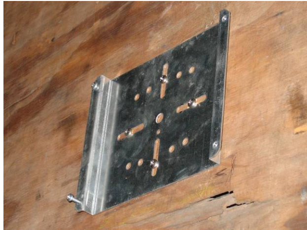
Figure 11: Antenna Mounting Bracket
