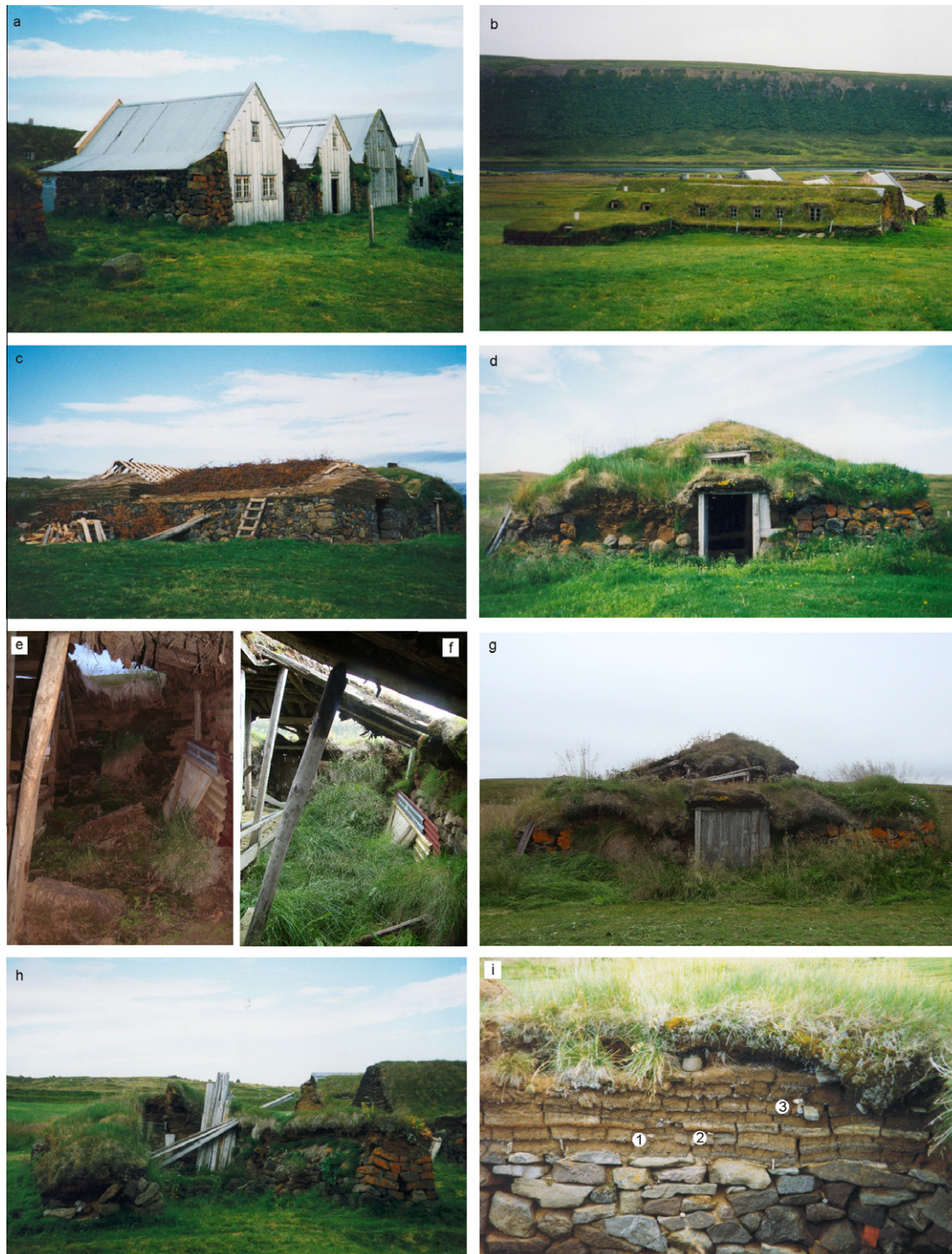
Fig. 2. Turf buildings at Thverá: (a) front of the main house; (b) back of the main house, showing light shafts protruding through the turf roof; (c) roofs of sheephouse 1 (right) and attached hay barn (left) under repair, showing turf strips being laid over a mat of birch brushwood; (d) sheephouse 2 in 1998, c. 40 years after it was abandoned, with an outer skin of stones beginning to peel away; (e) interior of sheephouse 2 in 2002, with the turf roof starting to collapse onto the floor; (f) interior of sheephouse 2 in 2010, with much of the roof collapsed, and the interior exposed to sunlight, rain, and soil formation processes; (g) sheephouse 2 in 2010, showing the collapsing roof, the progressive slumping of the stone and turf walls, and the living turf growing down over the exterior of the walls; (h) a storage building 70–80 years after abandonment, with a fully collapsed roof and slumping walls; (i) sheephouse 3 70–80 years after abandonment, showing shrinkage and cracking of the exposed turf being weathered by rain and frost; note the living turf overgrowing the top of the wall and the locations of bones (1, 3) and ceramics (2) protruding from the turf.
