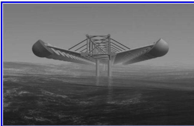
FIGURE 4.82 (See color insert following page 80.) WSE position in storm protection mode. (Courtesy of M. Kramer, “The wave energy converter: Wave Star, a multi point absorber system,” Technical Report, Aalborg University and Wave Star Energy, Bremerhaven, Denmark.)
