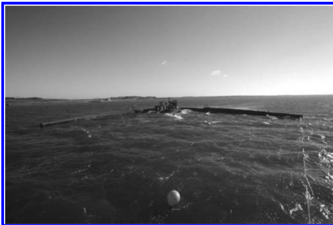
FIGURE 4.79 (See color insert following page 80.) Front view of the Wave Dragon with wave reflectors in the sides and the reservoir in the middle. (Courtesy of Wave Dragon ApS, available online at http://www.wavedragon.net/ )
