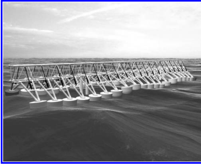
FIGURE 4.81 View of the WSE, a multipoint absorber. (Courtesy of M. Kramer, “The wave energy converter: Wave Star, a multi point absorber system,” Technical Report, Aalborg University and Wave Star Energy, Bremerhaven, Denmark.)
