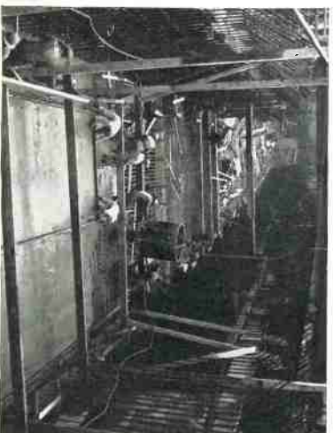
OPEN CUT IN BATTERY PARK
