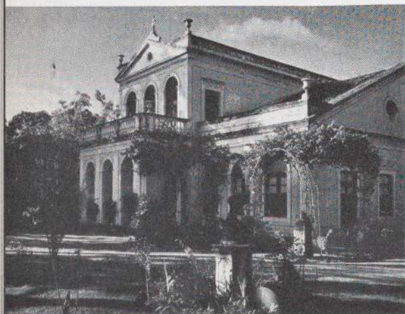
House of Senhora Donna Elvira Gonçalves de Moraes Avenida Rui Barbosa, 1596, Recife, Pernambuco, about 1850
