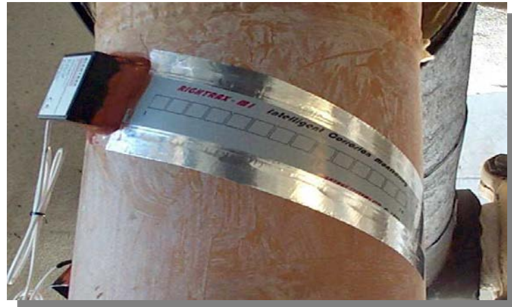
Hot Installation continuous @ 120 to 130 deg C prior to heat shield replacement
