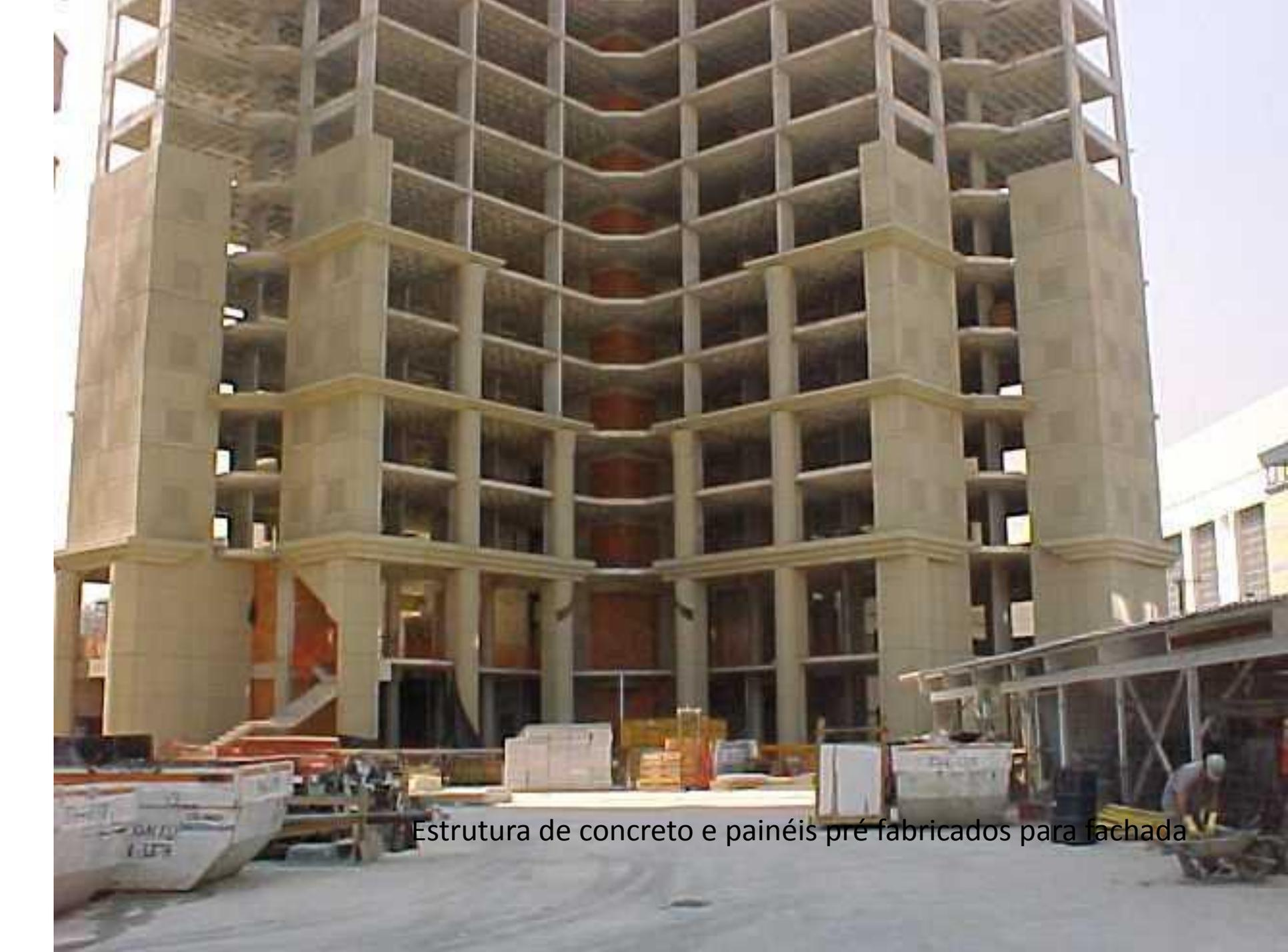
A tall building under construction, featuring a concrete frame and precast facade panels. The structure is composed of a grid of vertical columns and horizontal beams, with large, rectangular precast panels attached to the exterior. The building is situated in an urban environment, with other buildings visible in the background. The ground in the foreground is a construction site with various materials and equipment.
