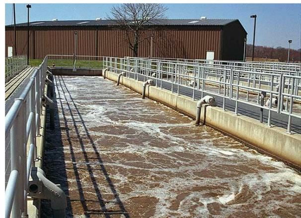
Fig.6. The bio-aeration tank<sup>16</sup>
