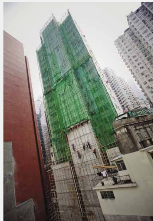
Workers assemble bamboo scaffolding on a skyscraper at a construction site in Hong Kong.
