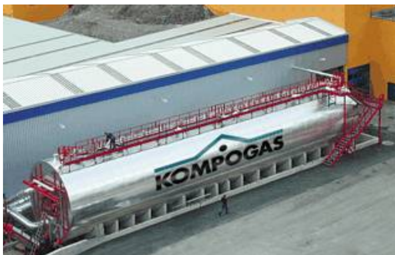
Figura 6 – Reator/digestor horizontal Kompogas
