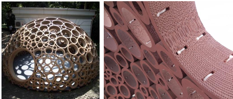
Figure 4.1. 10 Laminating technique for the curved packing structures with thin sheets
