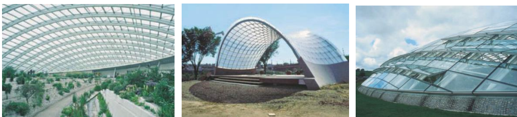
Figure 3.1.17 Integration of flat glass sheets in the spatial framework structures (Wurm, 2007)
