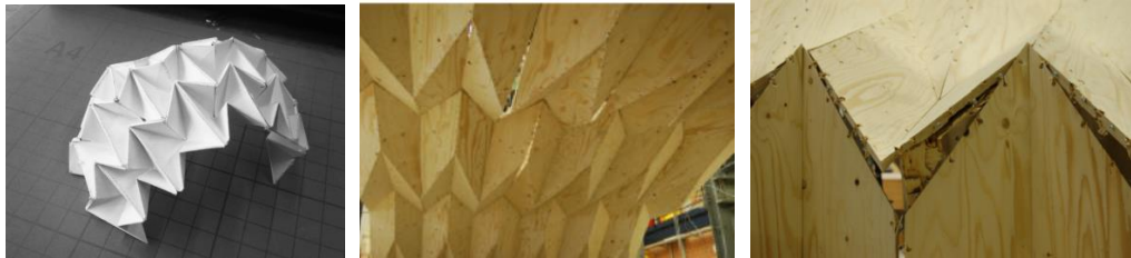
Figure 3.2.15 Folded Origami structure and joining details (Buri, 2010)
