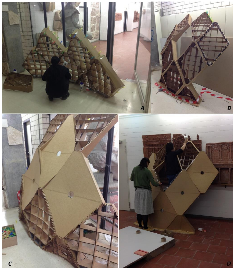
Figure 5.5. 13 Fabrication process of one cell groups in the bottom area by two people
