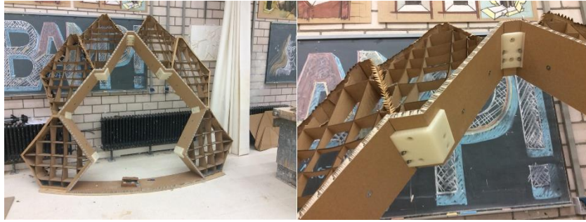
Figure 5.5. 14 Local stiffening for the entrance of the pavilion
