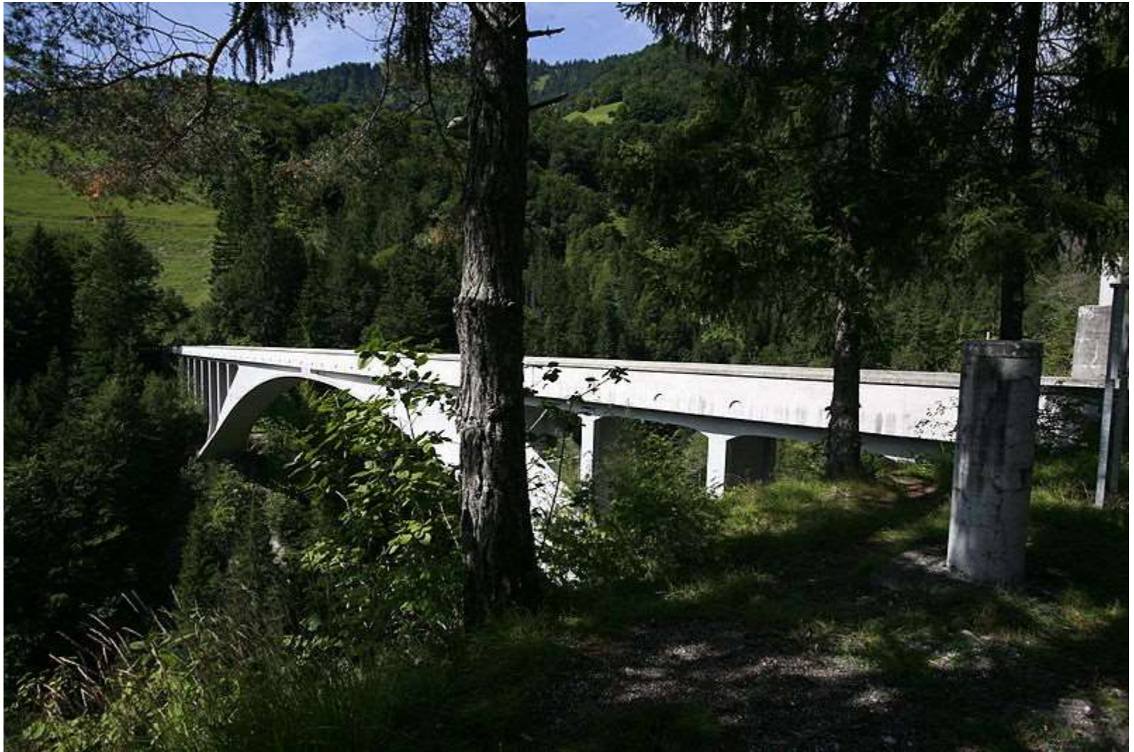
Ponte Salginatobel, Suíça Robert Maillart, 1929 (total length 133 metres, longest span 90 metres)
