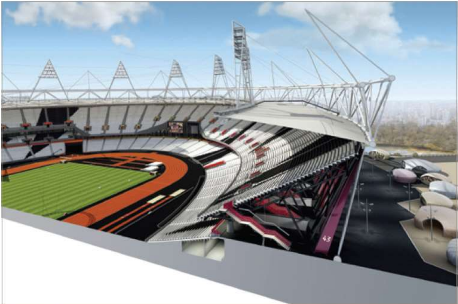
Figure 2. Typical stadium section showing permanent seating in lower concrete bowl, upper steel-framed temporary seating tier and external spectator facilities on podium
