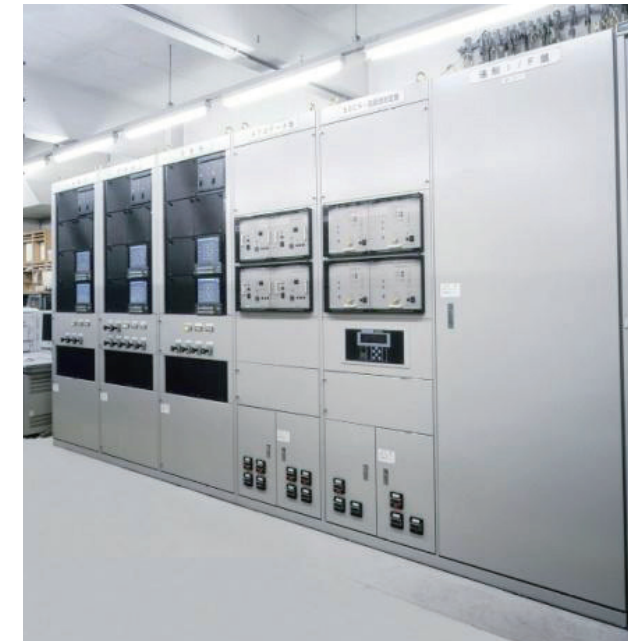
Control/Relay Panel
