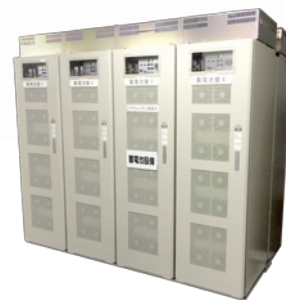
SCiB™ Traction Energy Storage System
