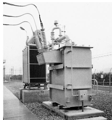
External view of AT (60/30 kV, 7500 kVA) (RTRI)
