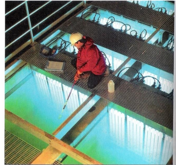
FIGURE 12.16 Ultraviolet light irradiates a thin layer of water, killing harmful organisms. (Flip Chalfant/The Image Bank/Getty)
