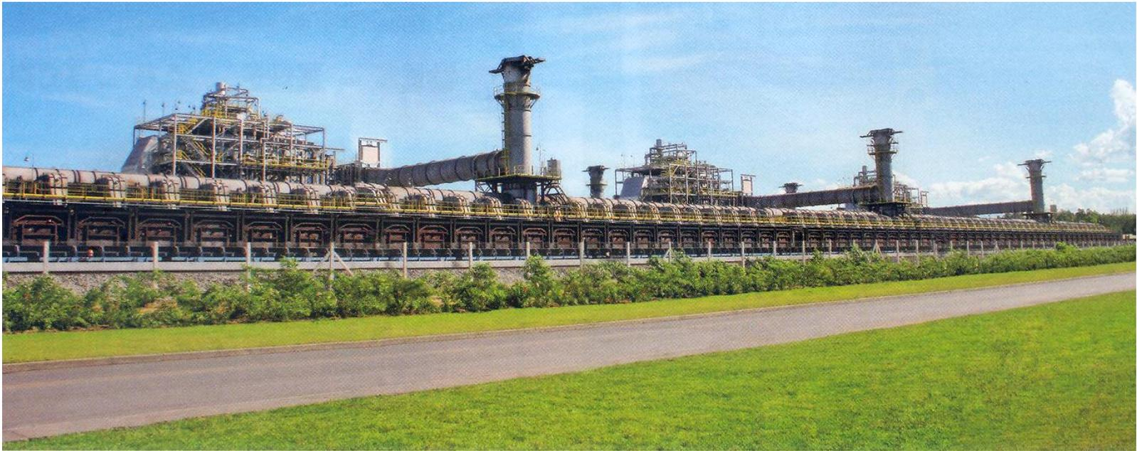
Coke oven battery with three heat-recovery boilers
