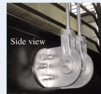
Side view of hanger rod and bracket (© Barry Goodno)
