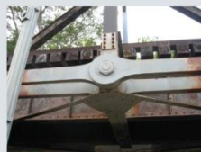
Pin connection on old bridge (© Barry Goodno)
