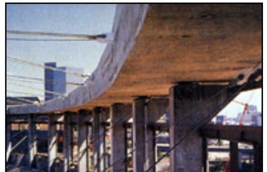
Fig. 4.6. "Georgia Dome" Detail of the compressed ring. Illustration taken from Setzer (1992)
