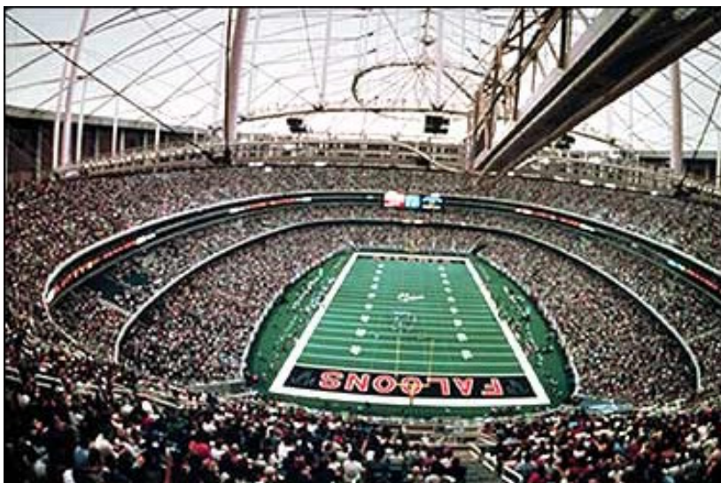
Fig. 4.5 "Georgia Dome" spanning 233.5x186m (by Weidlinger Asscts.) Illustration taken from Setzer (1992)
