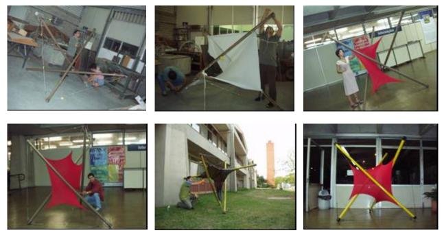
Figure 5. Several steps of the production of the MMF2
