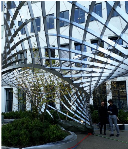
A gridshell composed of metal plates that run along asymptotic lines (lines of zero normal curvature) – TUM, 2017
