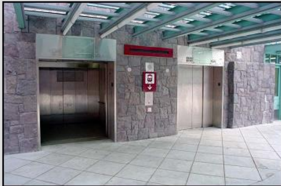
(a) Station Access (Portland, Oregon)
