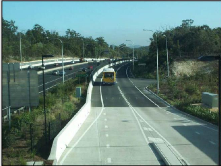
(a) Exclusive, Grade-Separated Facility
