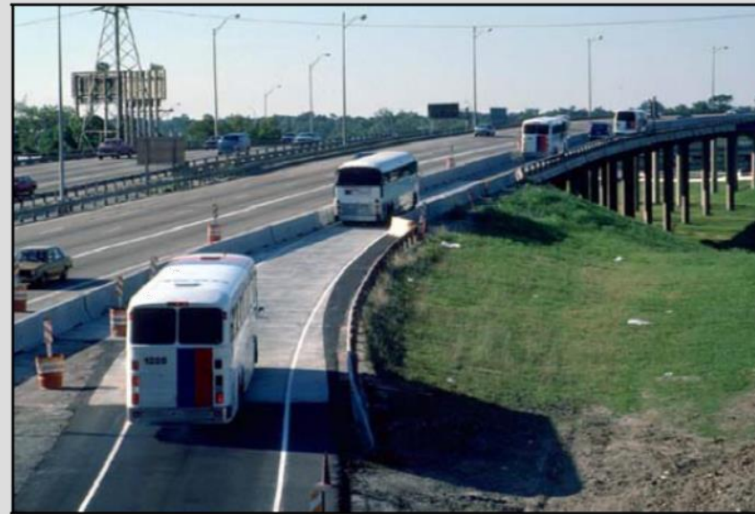
(b) I-45 North Freeway
