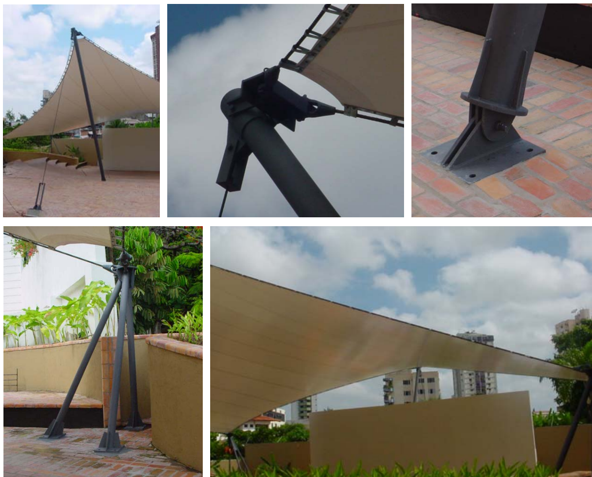
Figure 13. Some details of the MPBP membrane roof and anchorage system.
