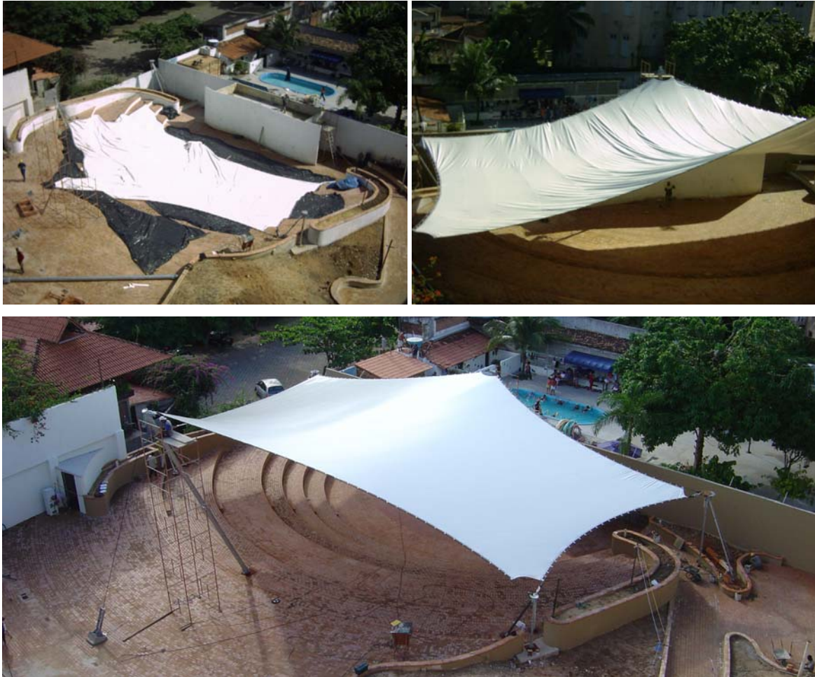
Figure 11. Three different stages of the assembling of the membrane roof of the MPBP.
