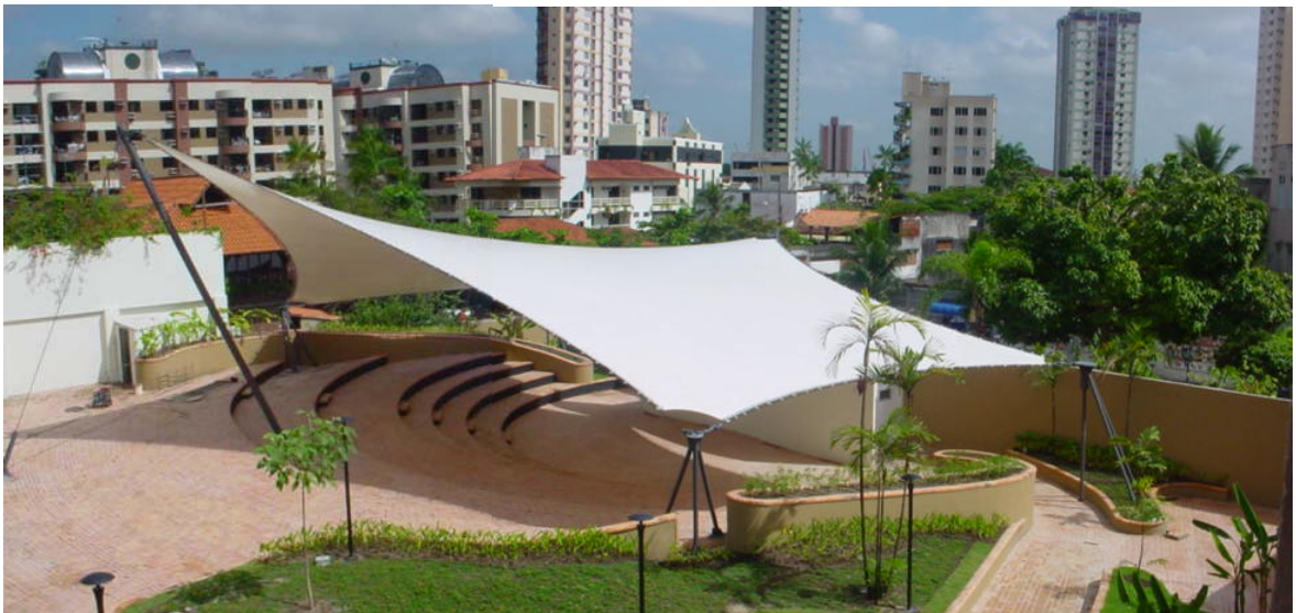
Figure 12. Final set up of the membrane roof of the MPBP, with the membrane completely taut.
