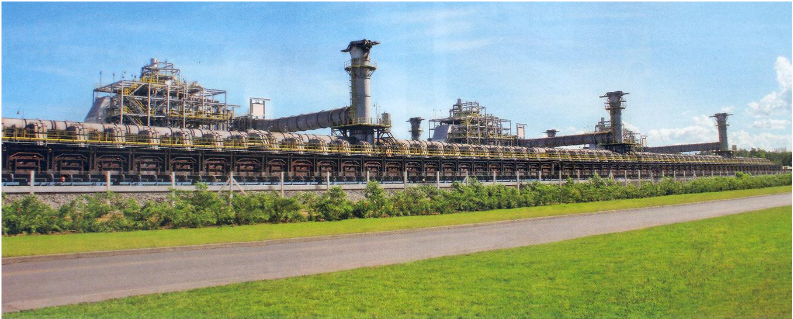
Coke oven battery with three heat-recovery boilers
