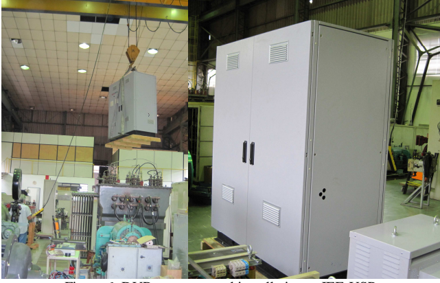
Figure 6: DVR transport and installation at IEE-USP.
