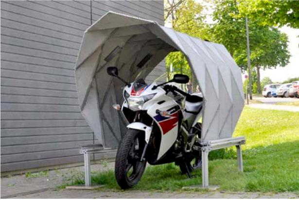
**Figure 19:** Oricrete bike shelter ('shell-ter' in [44]), designed and realized by researchers from RWTH Aachen [photo: Jan Dirk van der Woerd, RWTH Aachen], [44]
