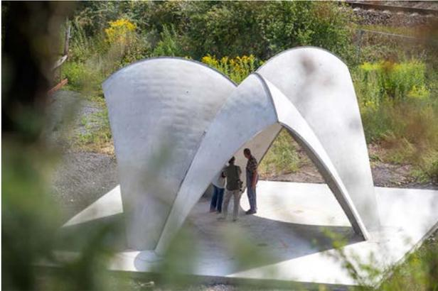
**Figure 11:** TRC structure made of six cast elements
