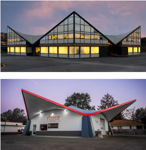
Figure 4: Pentagon Hall, London, UK, built c. 1960, and Auto Perfection car repair shop, Midland, MI, USA, built c. 1960-1962 (above: © Mike Deakin, below: CC BY 4.0 Ryan Collier)
