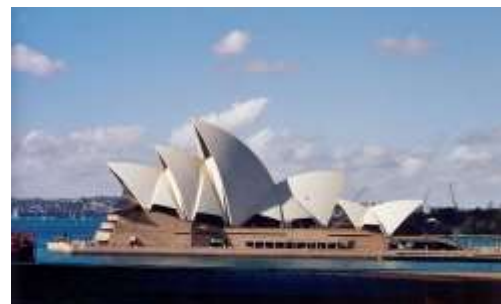
Sydney Opera House (1958 – 1973) Double thin shell ribbed ; Concept designer Jern Utzon; Architect E. H. Farmer , Peter Hall, David Littlemore, Lionel Todd ; Engineer: Ove Nyquist Arup
