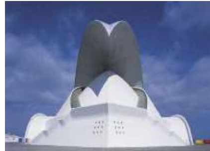
The all-concrete building is characterized by the dramatic sweep of its roof. Rising off the base like a crashing wave, the roof soars to a height of 56 meters over the main auditorium before curving downward and narrowing to a point. The building's plinth forms a public plaza covering the site and allows for changes in grade between the different levels of the adjacent roads.
