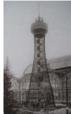
The world's first hyperboloid structure Vladimir Shukhov, Nizhny Novgorod, 1896
