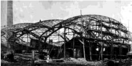
Vladimir Shukhov First double curvature diagonally framed shell during construction, in Vyksa near Nizhny Novgorod, 1897
