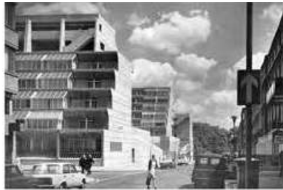
Fig. 8 South West side (Russel Square Underground Station view )
