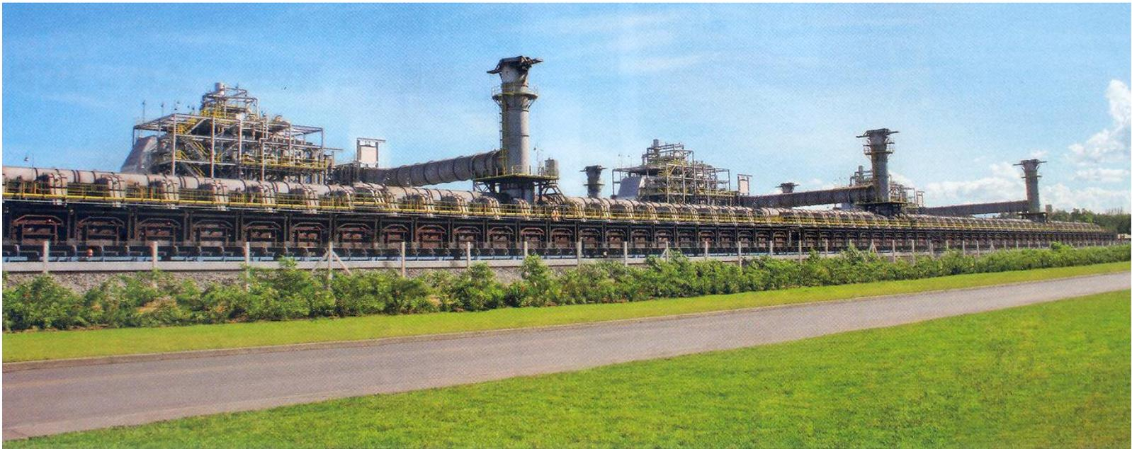
Coke oven battery with three heat-recovery boilers
